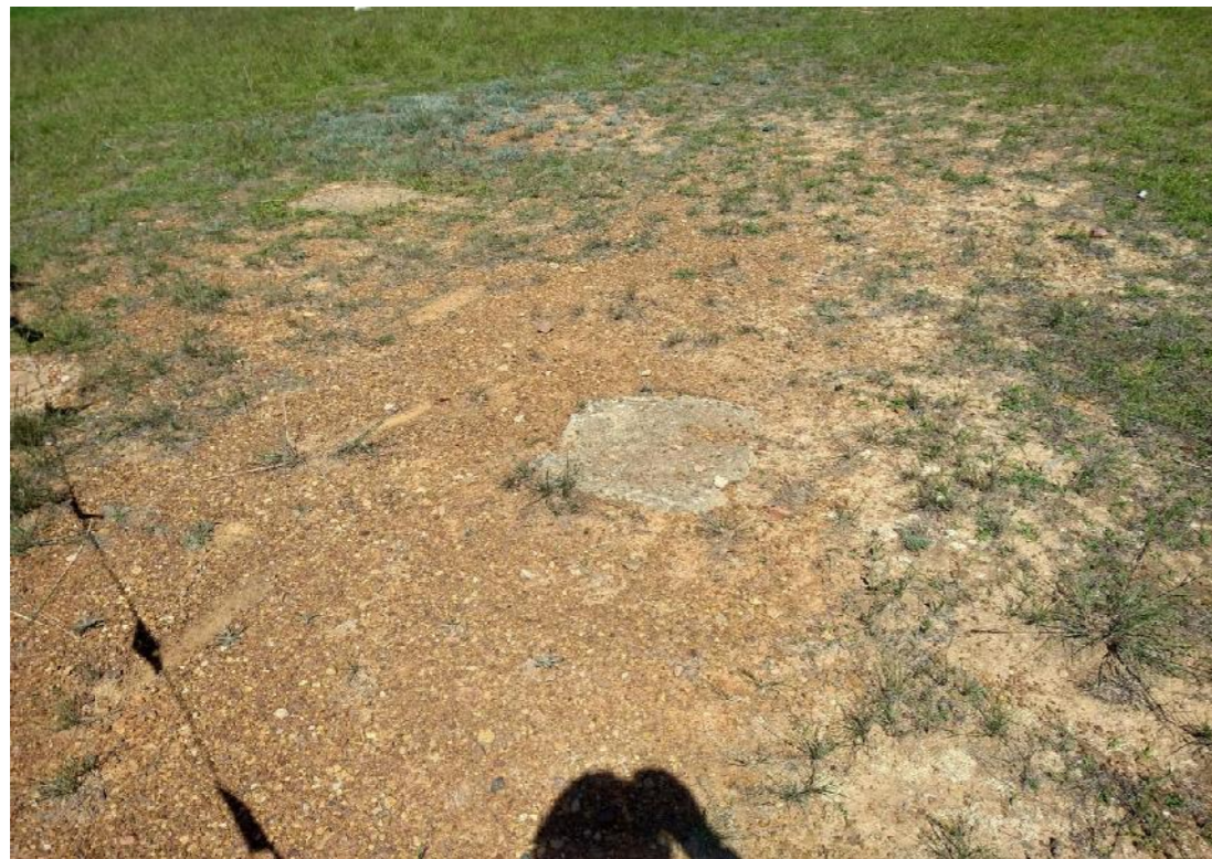
Photo 3: Concrete footings observed in north western corner of the site.
